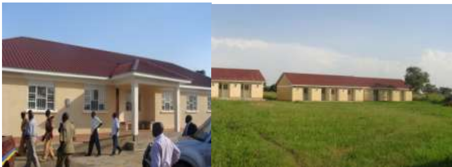
Figure 2 Amolator Police station and Barracks
