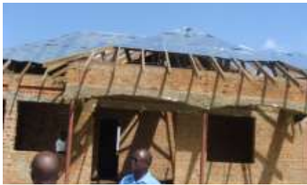
Figure 6: Amolator DPP offices financed in 2006/7 is just being roofed in 2010
