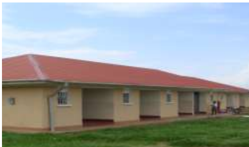
Figure 9 Pader Police barracks completed in 2008 and still unoccupied
